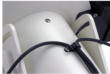
Installed Cable Clip
